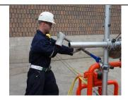
All the nuts on the universal clamps holding the cross arm where the drill is mounted to the two upright column bars must be tightened as much as possible. The operator should have a three foot length of pipe that fits over the handle of the chuck wrench so that maximum leverage can be exerted to tighten the nuts on these universal clamps.
